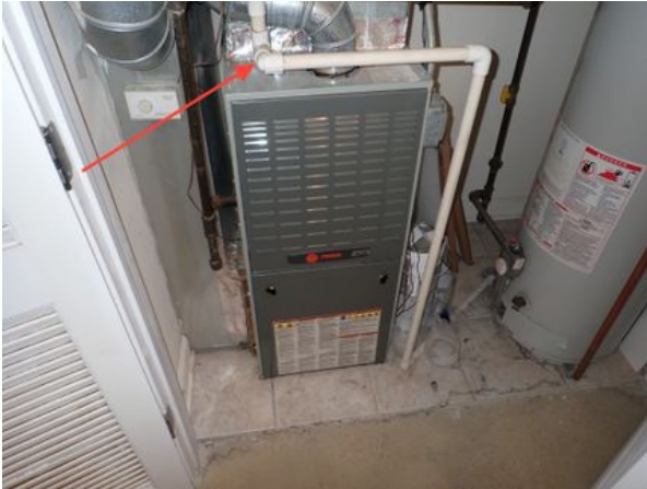
Condensate Drain on Furnace
