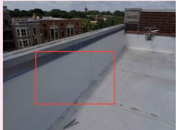
Front Parapet Wall Covered
