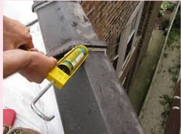
Clay Tile Caulking Example
