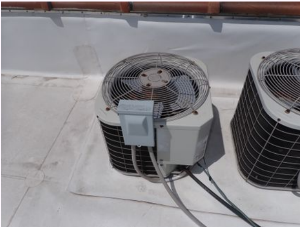
Older A/C Unit
