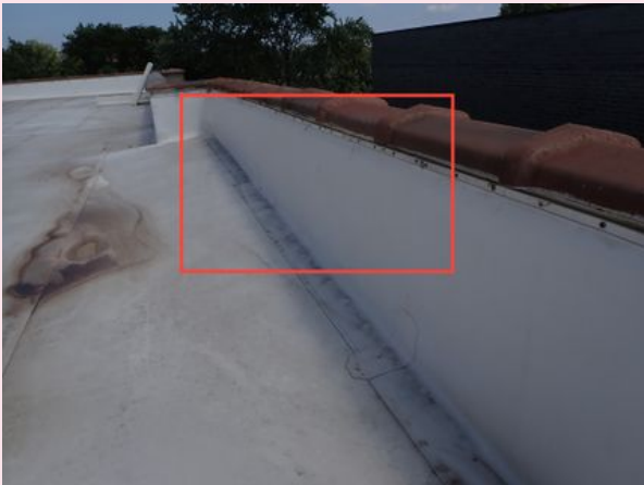
Parapet Walls Covered
