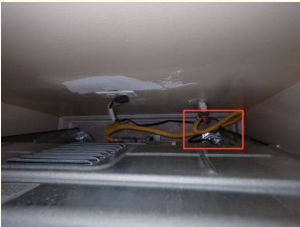
Missing or Ineffective Anti-tip Device
