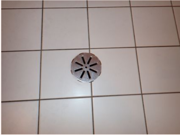
Floor Drain in Bathroom
