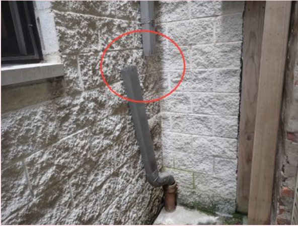
Disconnected Downspout
