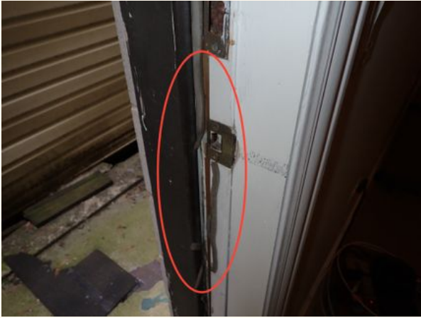
Missing Weatherstripping
