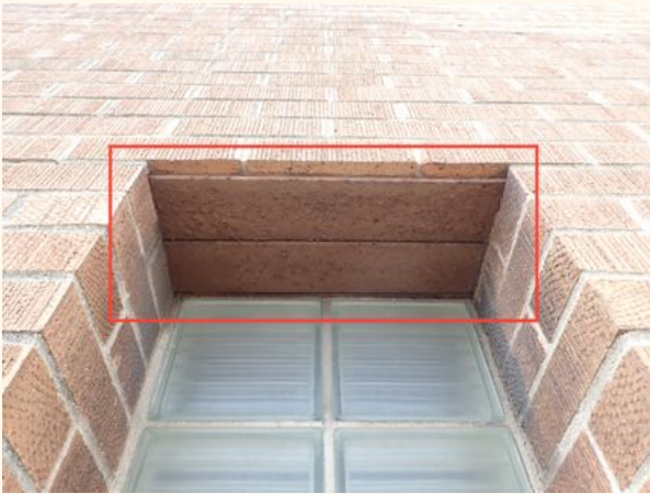
Corroding Paint on Lintels
