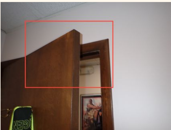
Door on Office Hitting Doorframe
