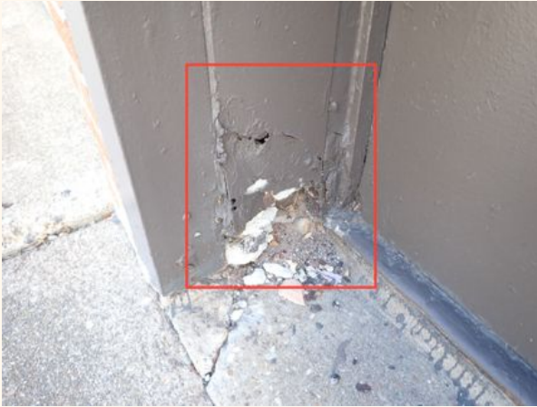
Deteriorated Doorframes
