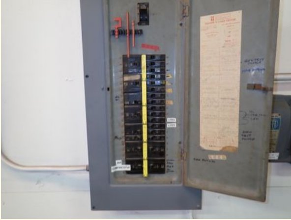
Full Panels in Shop Area
