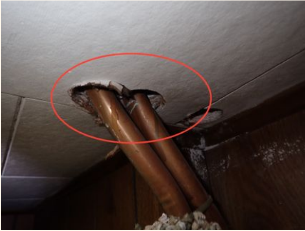
Older Ceiling Panels
