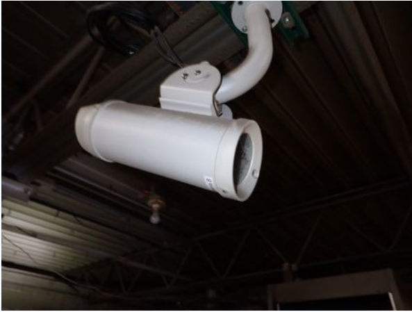
Low Voltage Surveillance Equipment
