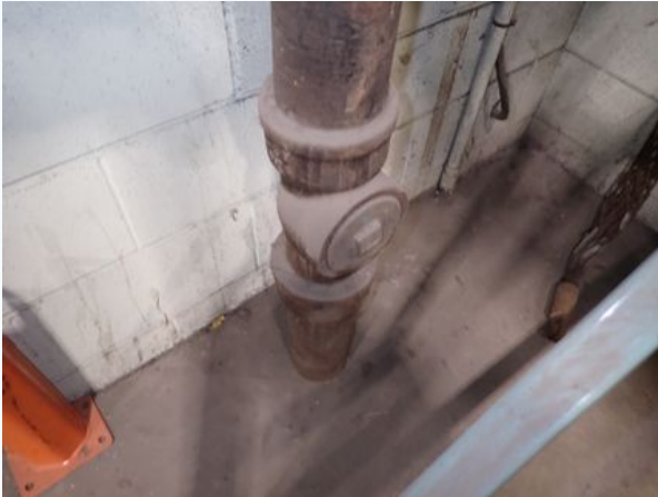
Clean-out in Shop Area
