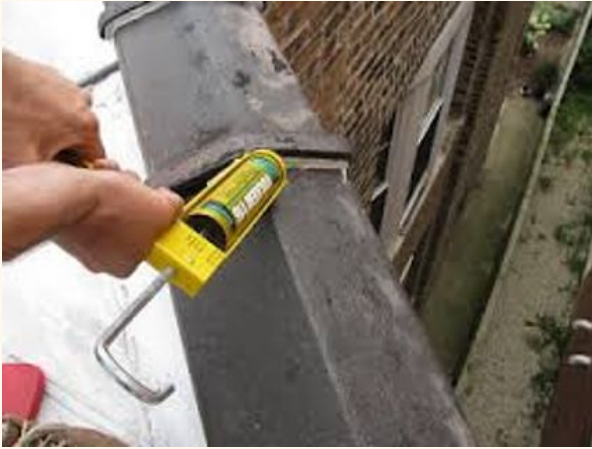
Clay Tile Caulking Example
