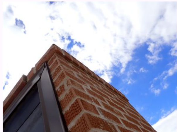
Recent Re-pointing on Chimney
