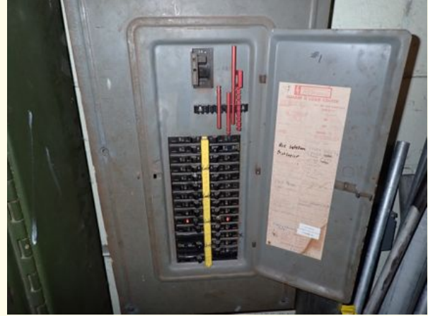
Full Panels in Shop Area
