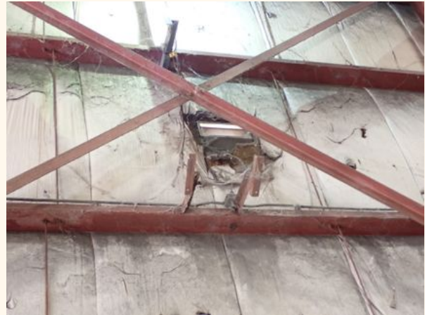
Open Vents on Interior
