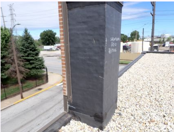
Chimney Covered with Roofing
