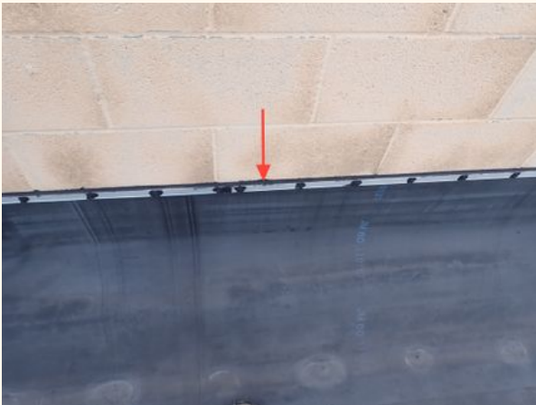
Termination Bar Flashing on Walls
