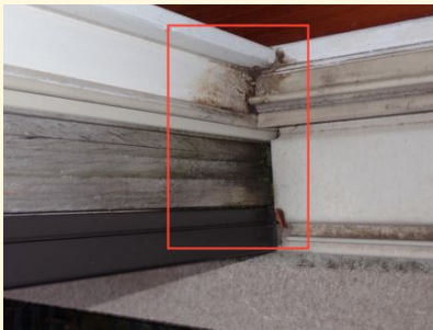
Deteriorated Doorframe
