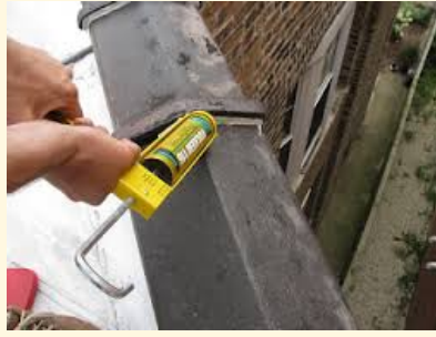
Clay Tile Caulking Example
