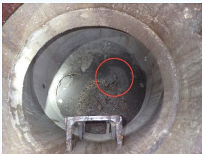
Drainage Location in Manhole
