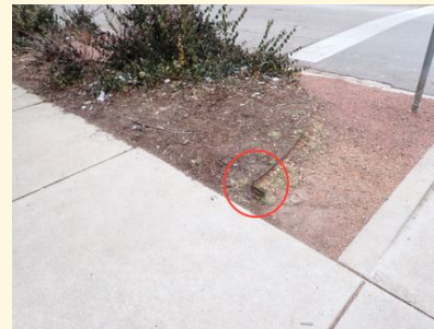
Exposed Metal Edging
