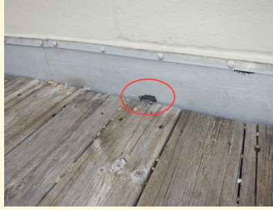
Damaged Roofing
