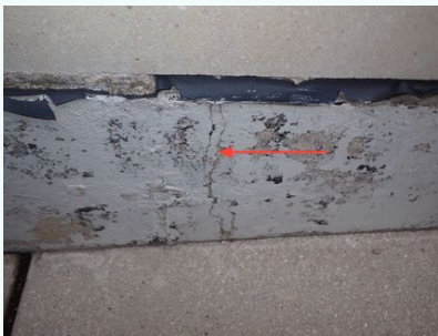
Foundation Crack
