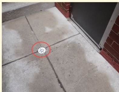
Small Drains by Lower Level Entry Doors
