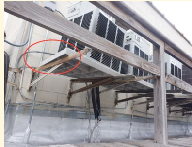
Base Balancing on Brackets
