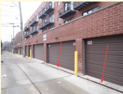
Trench Drains by Garages
