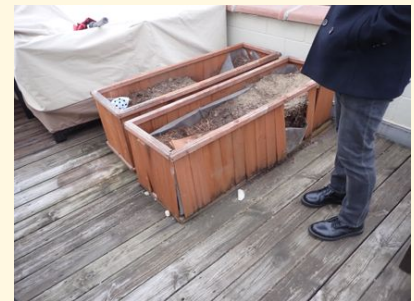
Deteriorating Planters on Roof
