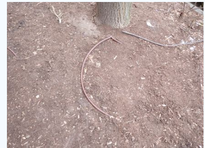
Exposed Irrigation Components
