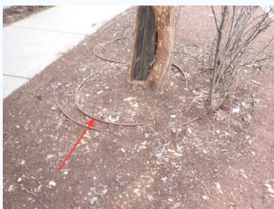
Exposed Irrigation Components
