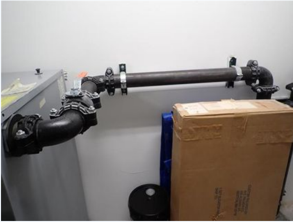
No Leakage Observed on Visible Elevator Piping
