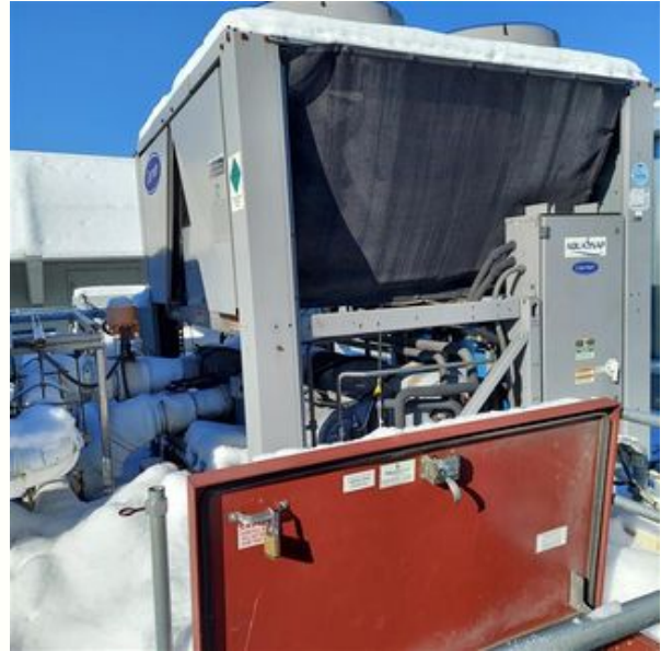
Carrier Air Cooled Chiller
