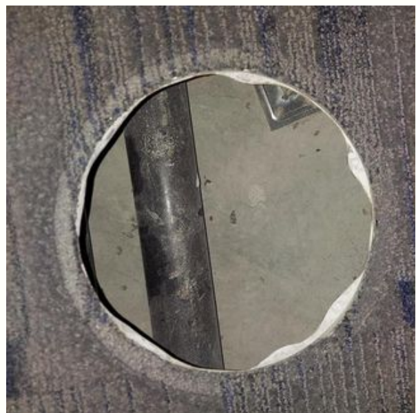
Underfloor Plenum System
