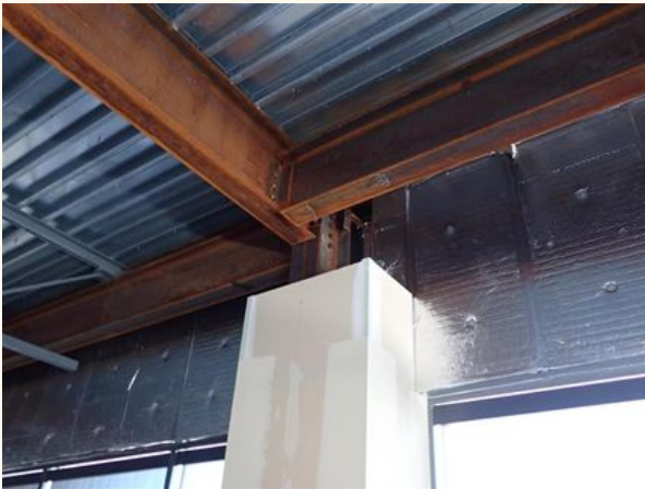
Column to Beam Connection on Fourth Floor
