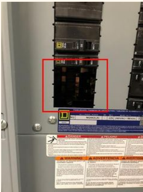
Open Twist-outs on Panel 3 rp-1
