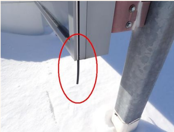
Loose Rubber Gasket
