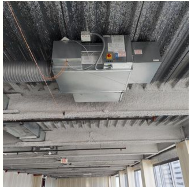
Typical Ceiling Mounted Fan Powered VAV box
