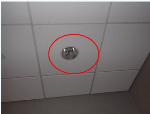
Numerous Ceiling Fixtures
