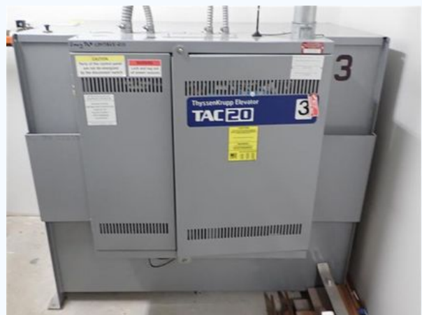
Hydraulic Elevator Units
