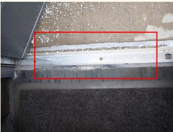
Deteriorated Threshold
