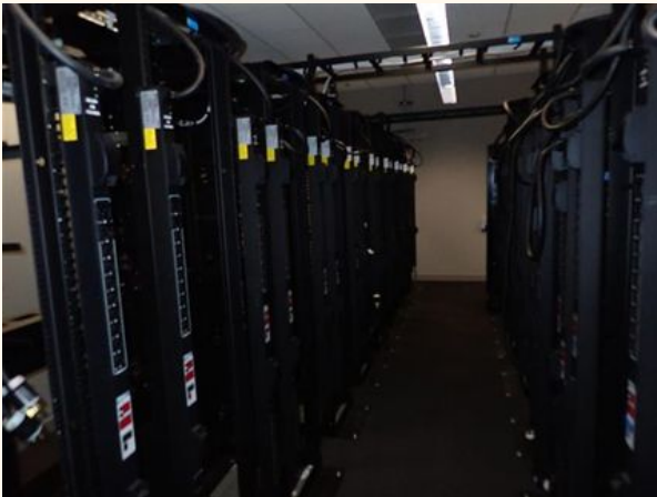
Former Server Racks
