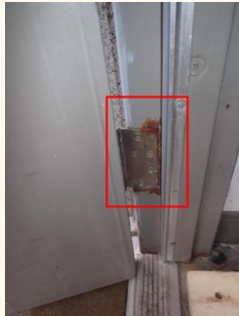
Corroded Hinges
