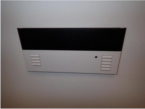
Low Voltage Alarm System
