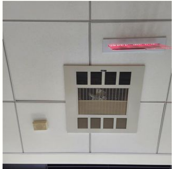
Electric Ceiling Heater
