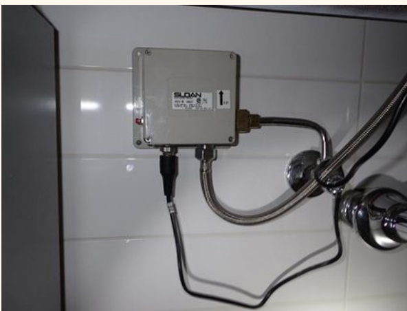
Battery Operated Sink Controls
