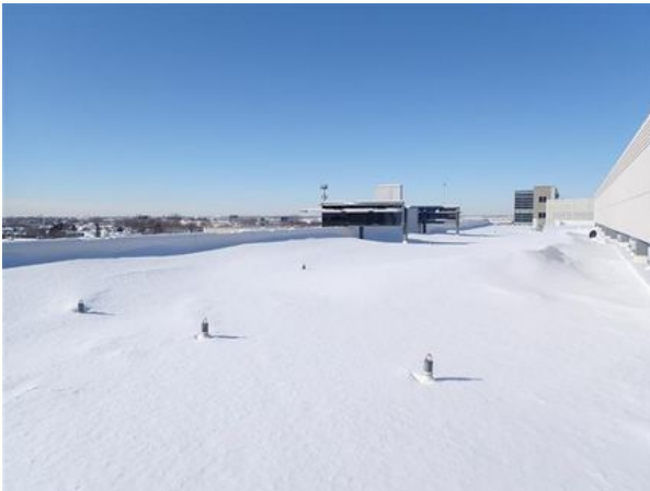
Roof Covered With Snow
