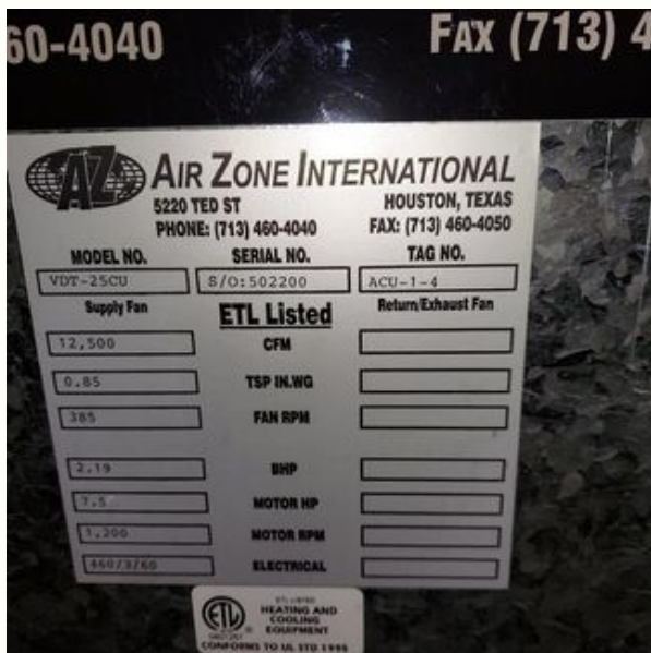
Air Column Unit Data Plate
