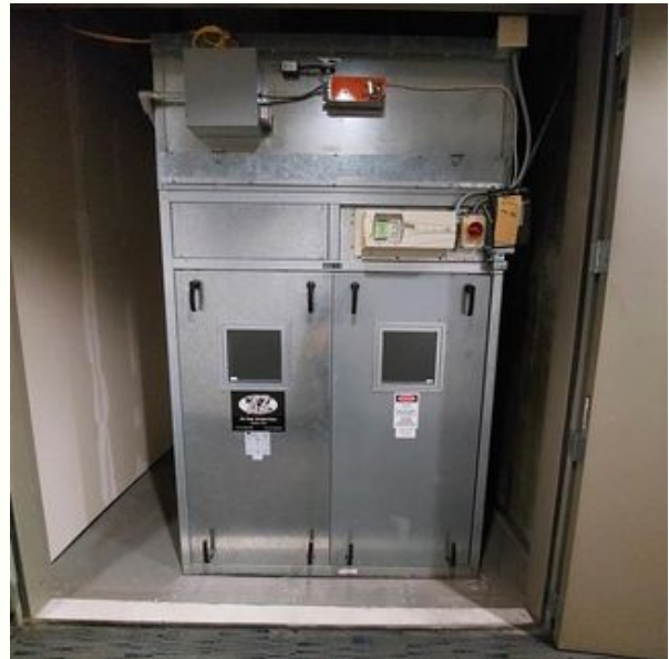
Typical Air Column Unit
