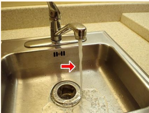
Residual Flow in Some Fixtures
