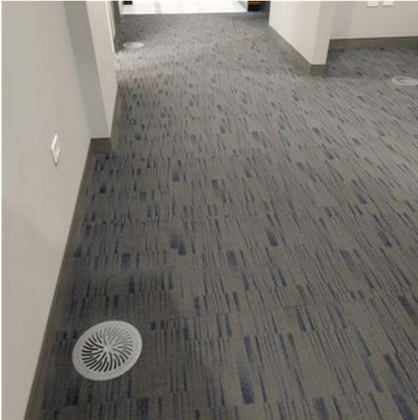
Typical 8" Floor Diffusers
