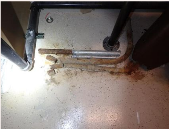
Unknown Deteriorated Components Replaced
