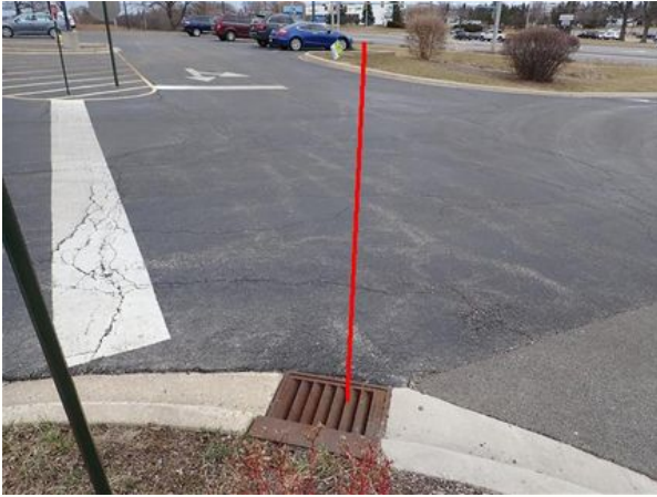
Storm Sewer Across West Drive
