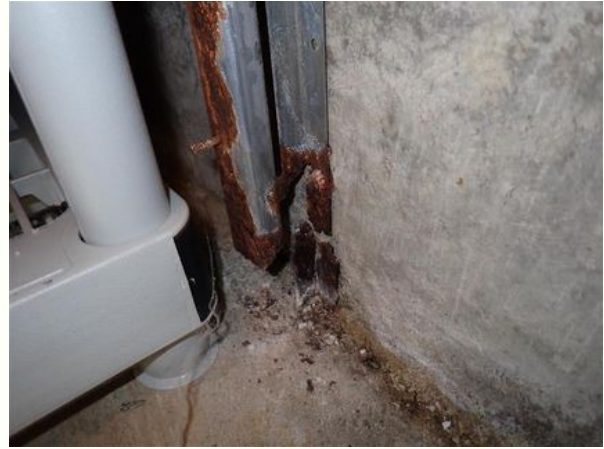
Corroded Framing
