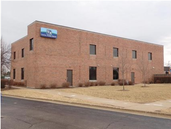
Grading Sloping Away from Structure
