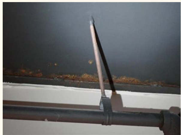
Corrosion in Metal Landing by Door
