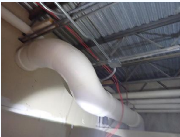
Visible Pans and Trusses Between Floors
