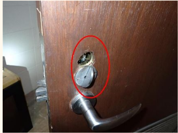
Hole by Lock Mechanism
