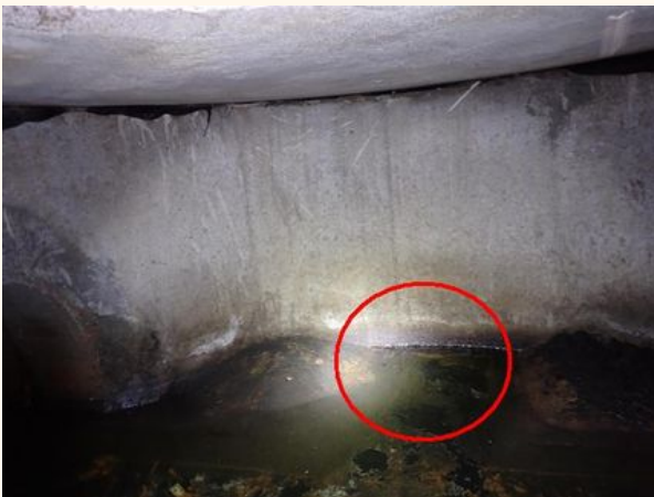
Possible Discharge Pipe in Manhole by Grand Ave
