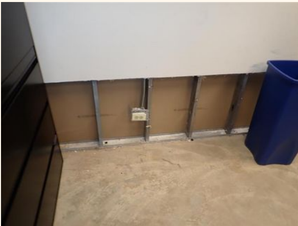
Walls Removed in Storage Area
