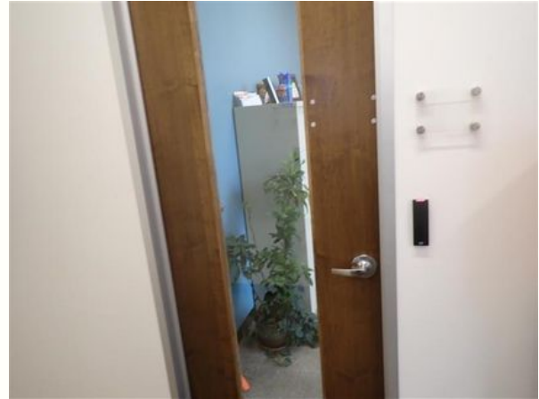
No Access to Insurance Office
