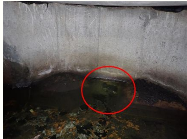
Possible Pipe Location in Manhole by Street
