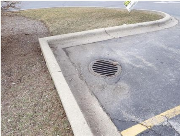
Manhole in Corner of Lot
