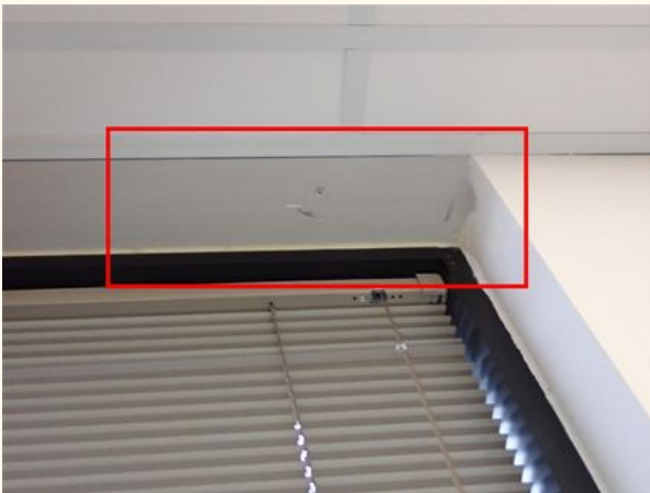
Potential Repaired Window Areas
