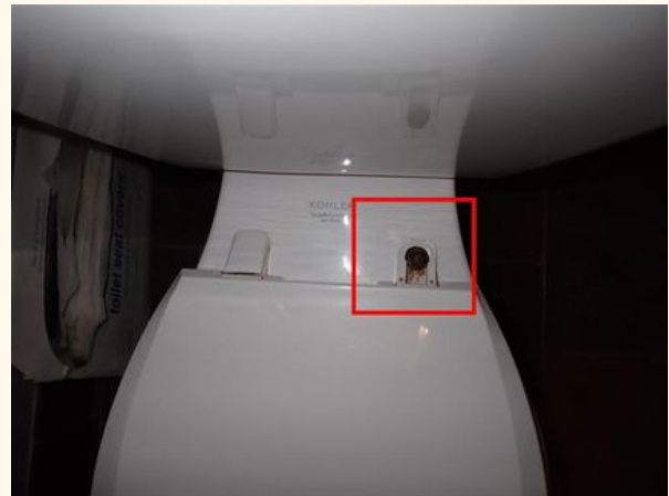
Missing Cap on Toilet Seat
