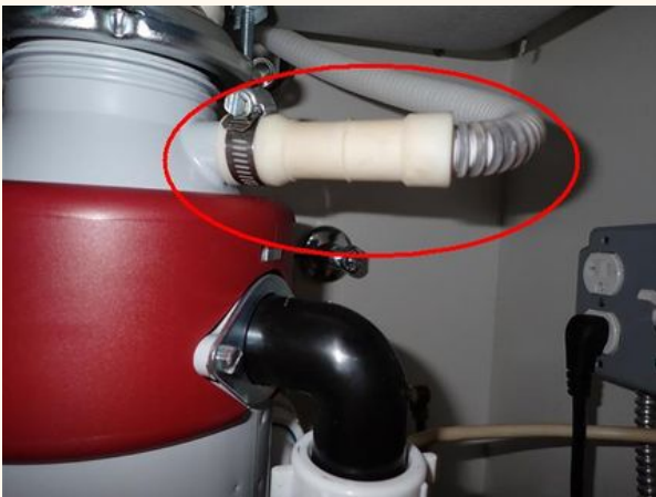
Dishwasher Connected to Food Waste Disposer
