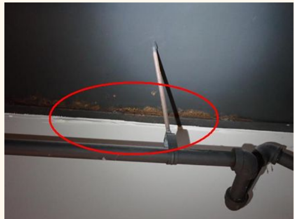
Corrosion on First Floor Stair Landing in NE Corner Stairwell
