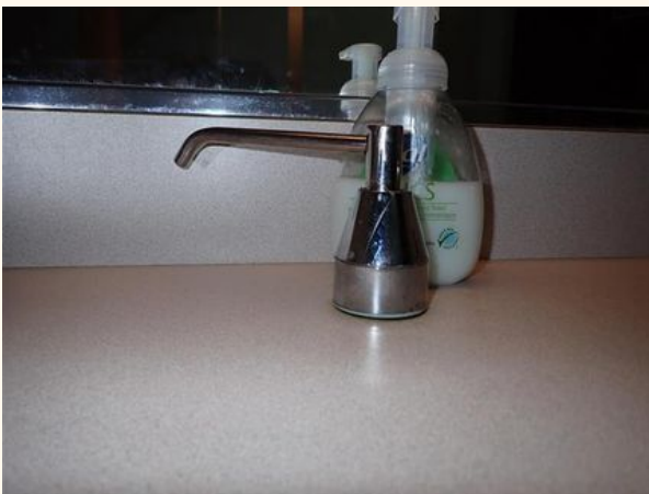
Non-functional Soap Dispensers
