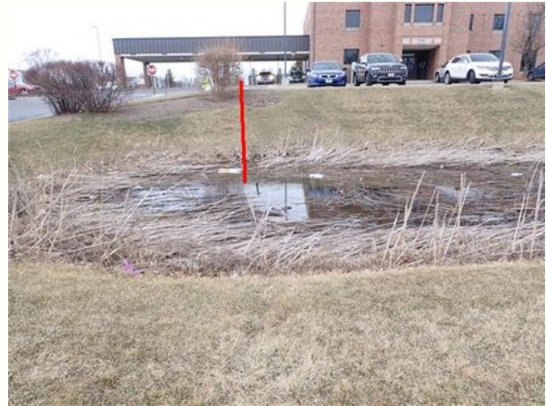
Storm Sewer From Manhole into Pond
