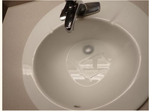
Standing Water in Sink
