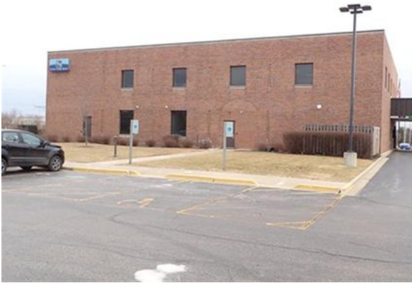
No Significant Cracking in Exterior Masonry Walls
