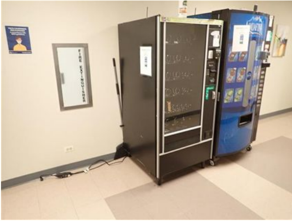
Unplugged Vending Machines in Basement
