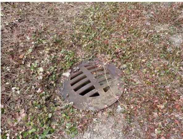
Large Drain in Garden Area
