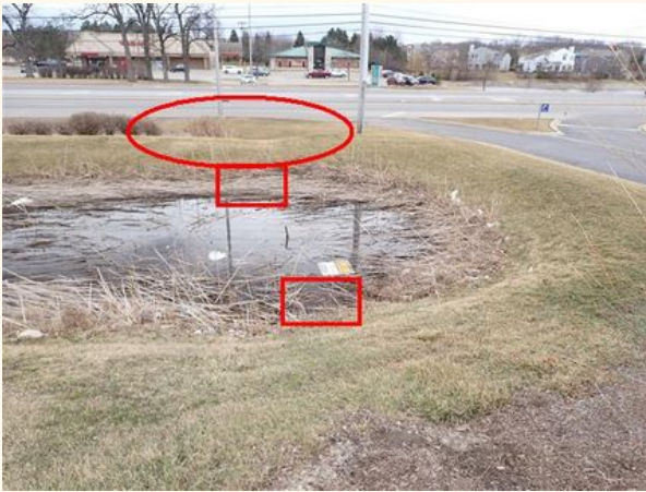
Basin Overflow Low Spot and Presumed Inlet and Outlet for Pond
