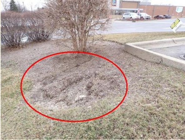
Eroding Areas Around Trees
