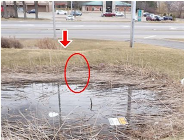
Manhole By Street - Presumed Pipe From Pond
